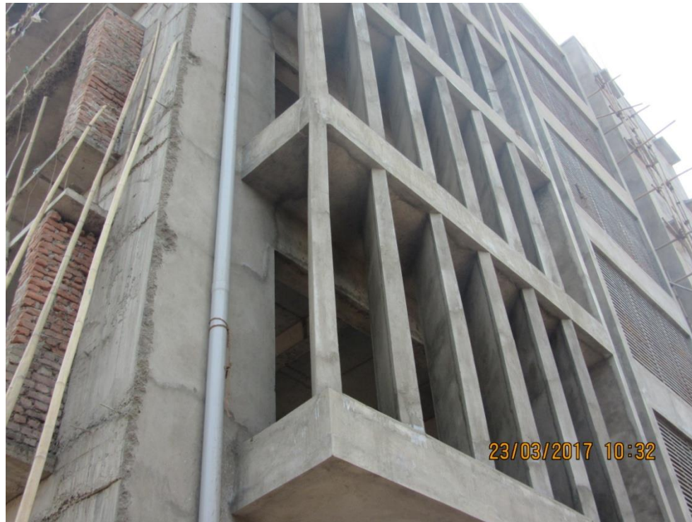
Fig: Construction Site and Surroundings
