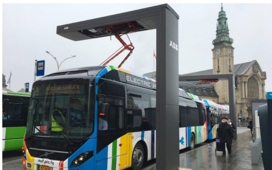
FIGURE 7: DC PANTOGRAPH CHARGING OF E-BUS USING AN OFF-BOARD BOTTOM-DOWN ARRANGEMENT IN LUXEMBOURG [SOURCE: (KYLE, 2017)]
