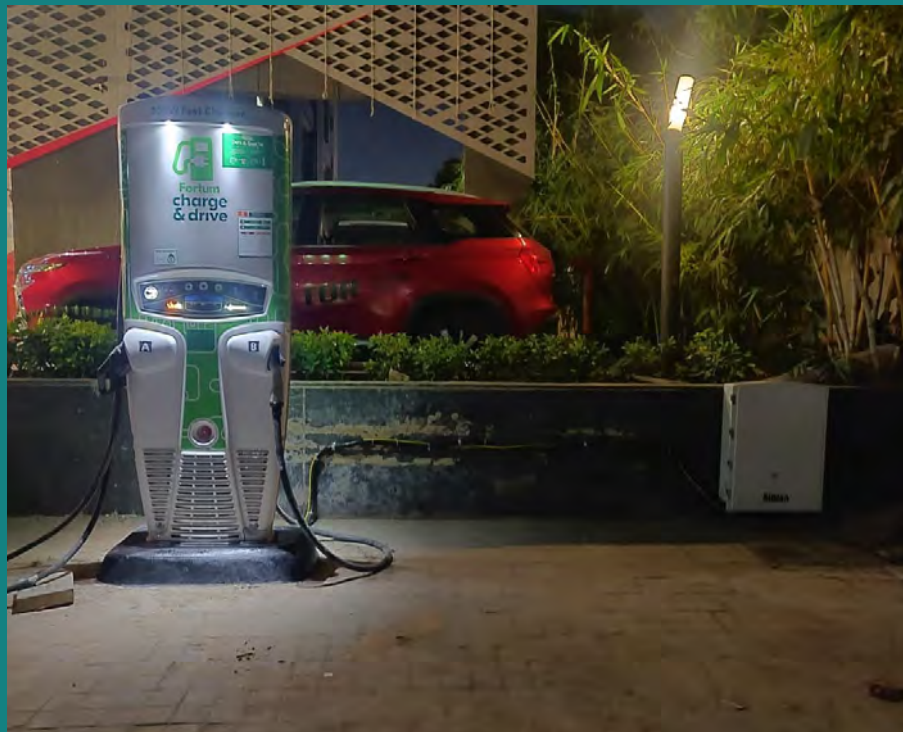
FIGURE 20: 50 KW DC CHARGER IN AHMEDABAD
