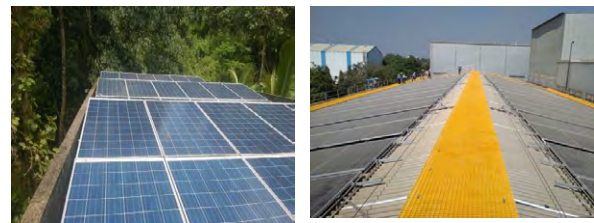
Figure 3: Power plant with (a) No access to far end PV arrays, (b) proper walkways for accessing PV arrays
