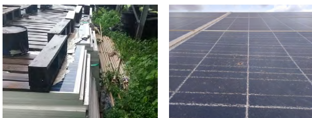
Figure 8: Faulty PV panels in a 6 year old utility scale power plant
