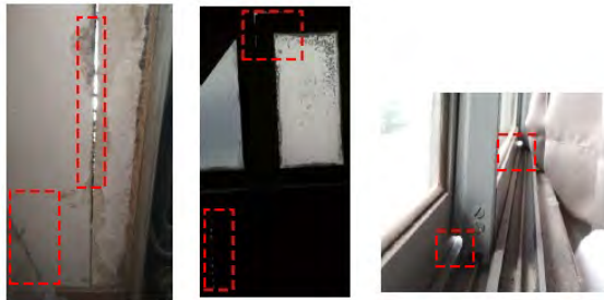
Figure 8 Leakage pathways through window perimeter
