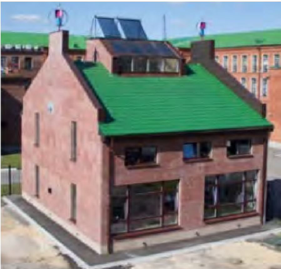
Figure 14: View of the Celver House in Nizhny Novgorod, Russia. Source: (Green Building Council Russia, 2012)
