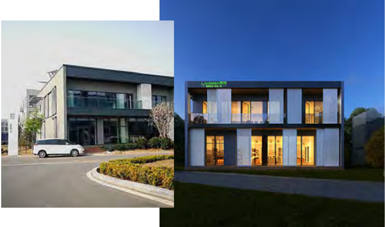
Figure 8: Views of Passive house in Beijing, China. Source: (Database, 2017)
