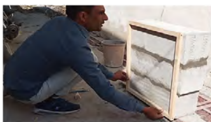
Step 7: Wood framing to hold insulation layer on AAC Blocks
