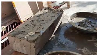
Step 3: 5-10 mm AAC Block ADHESIVE by Laticrete
