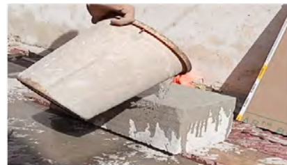
Step 2: Curing AAC Block
