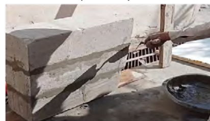
Step 6: Fill grooves between AAC Blocks
