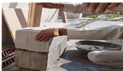
Step 5: Proper alignment of AAC Block
