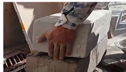
Step 4: Place the another AAC Block and repeat the process
