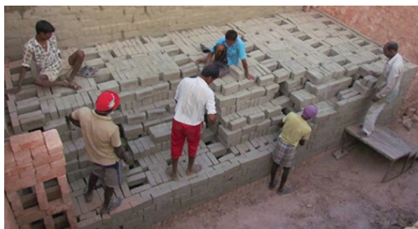
Figure 14: Dense single Zig Zag brick setting
