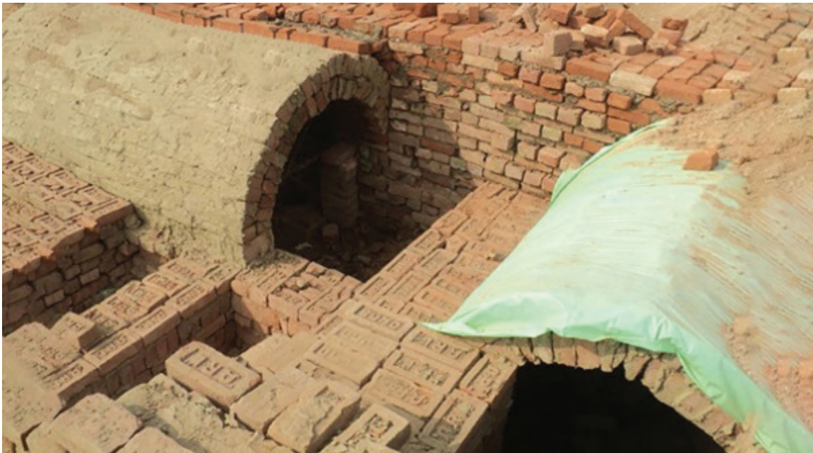
Figure 8: Central duct arch covered with plastic sheet (
