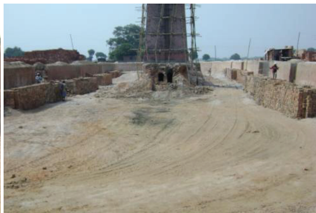
Figure 6: Safe storage of bricks
