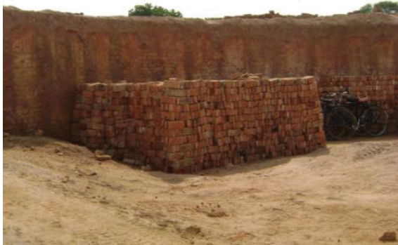
Figure 7: Demolition of Miyana
