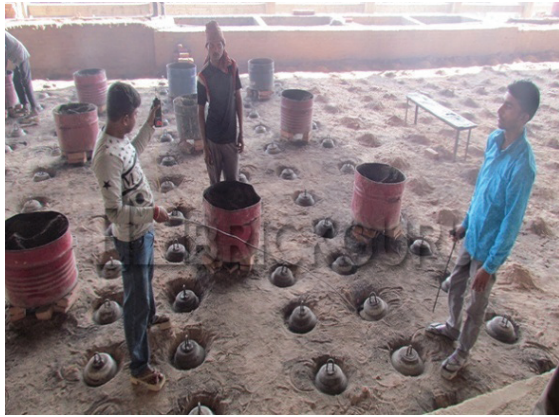
Figure 45 Temperature measurement in brick setting
