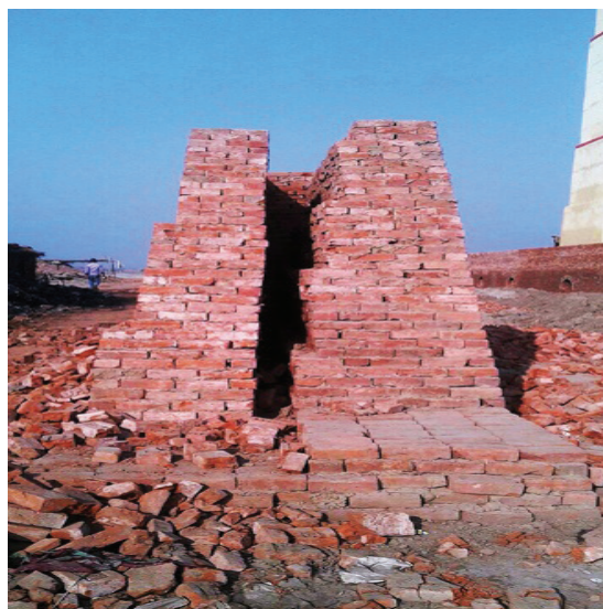
Figure 10: Outside wall of the kiln stepped on the outside
