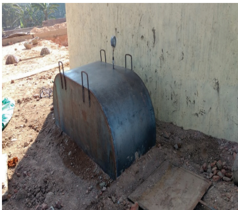
Figure 47 Flue gas temperature measurement on shunt
